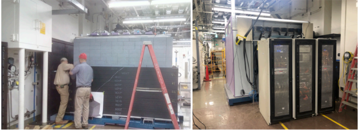
Figure 4.24: (left) Layers of lead (gray) and BPE (black) shielding installed on the exterior of the detector package by HFIR workers. (right) Electronics racks after components were installed and cables connecting to the feedthrough bulkhead panels.
